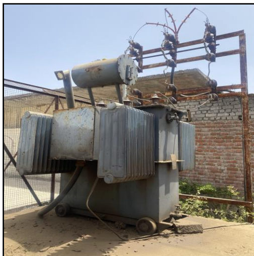
Figure 2.1:- 11 kV Feeder and 630 kVA and 500 kVA
