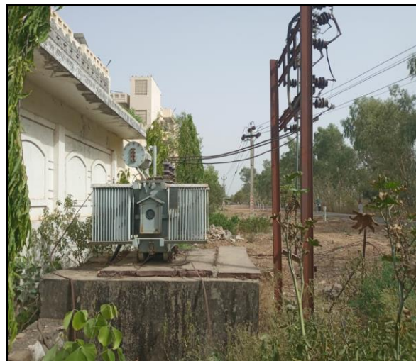
Figure 2.1:- 11 kV Feeder and 630 kVA and 500 kVA
